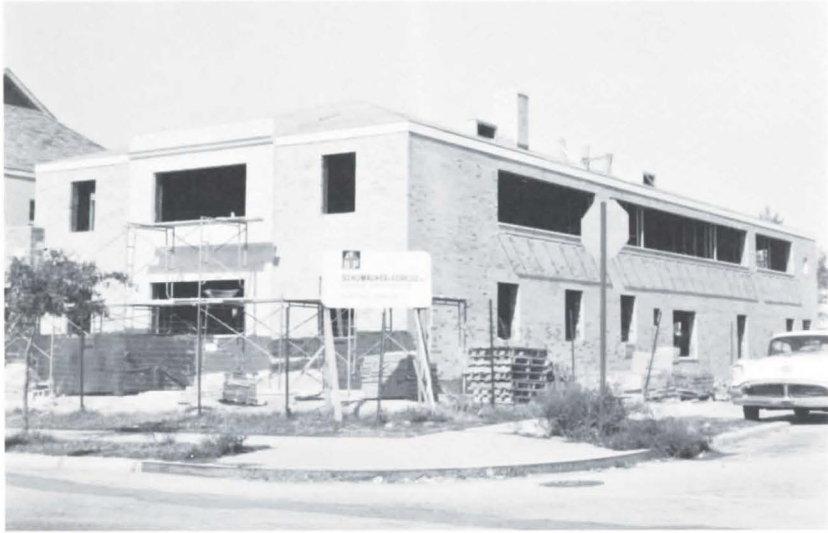
CONSTRUCTION OF SCHOOL AND COMMUNITY CENTER
