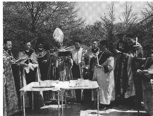
Blessing of Foundation Stones 1965
