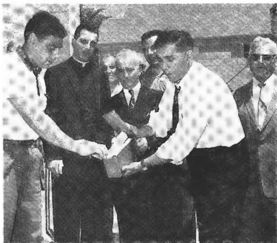
Placing historical church documents in corner-stone.
