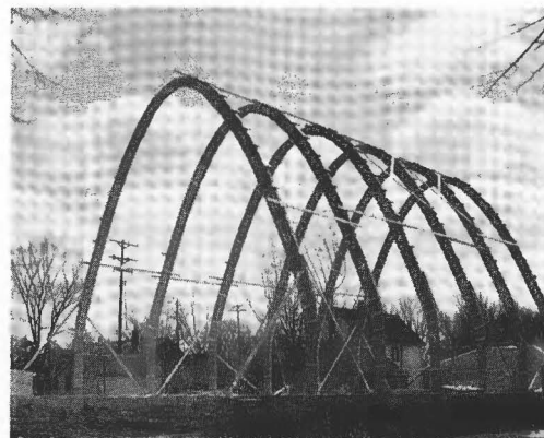
Work proceeds on schedule and the parabolic arches of the modern Byzantine design are erected in the Spring of 1961.
