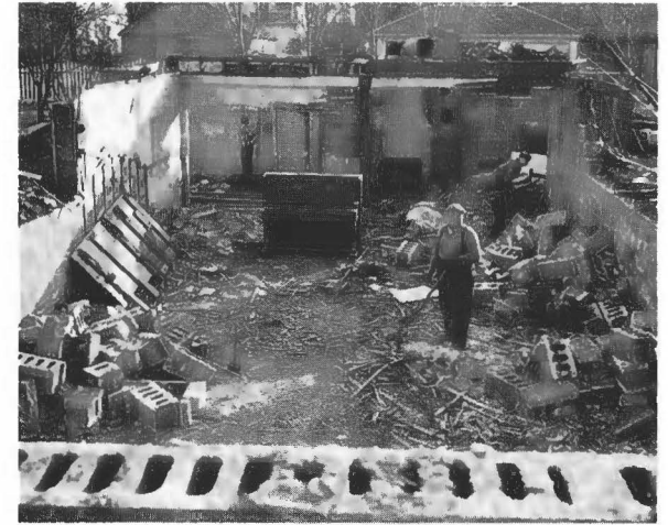
The piano still stands on firm footing as workmen proceed with demolition of the fire ruined structure in November 1960 — first phase of constructing a new church.
