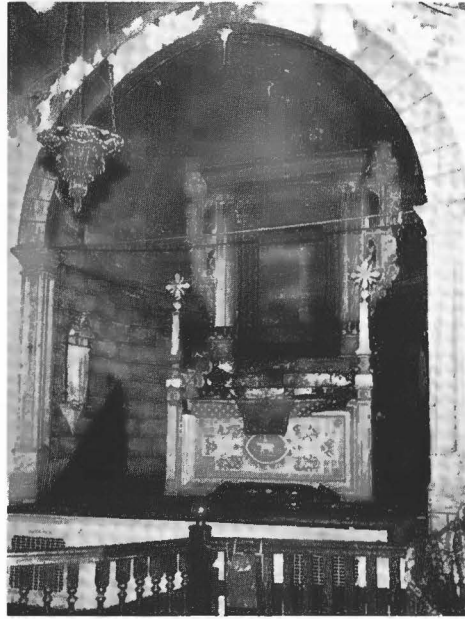
Tragedy struck in February, 1960, when fire gutted the church and destroyed the altar.
